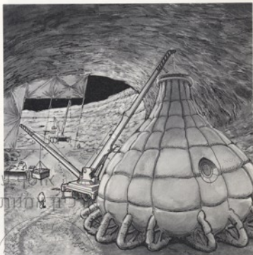
Self-supporting inflatable being erected in a lava tube.
